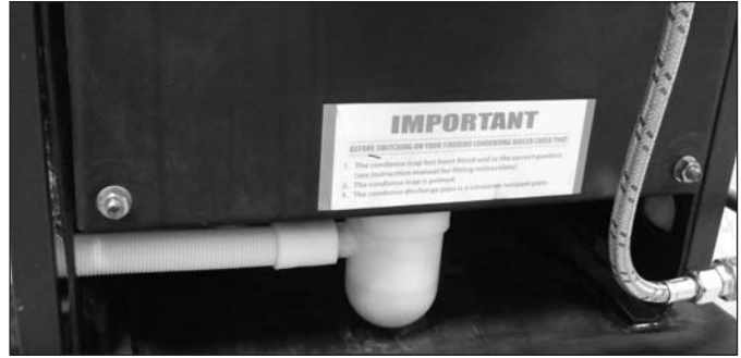
The condensate trap is located at the base of the boiler
